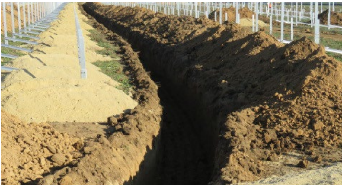
Figure 4: Trench for underground cabling
