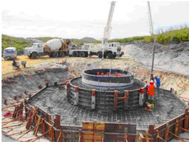
**Figure 3-2. Construction of Typical Spread Footing Foundation.**
